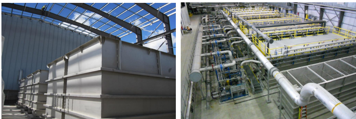
Figure 2: Stainless steel membrane tanks
