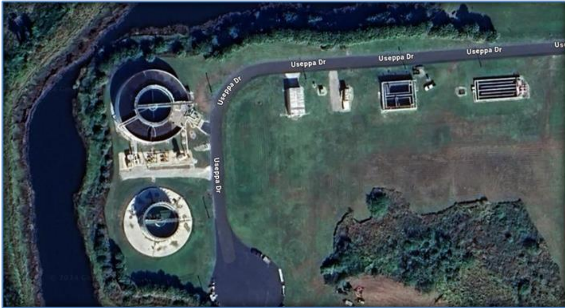
Figure 10 – Example Installation (Ave Maria WWTP)
