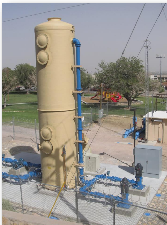
Figure 7 – Packed Tower Aeration (H2K Technologies)
